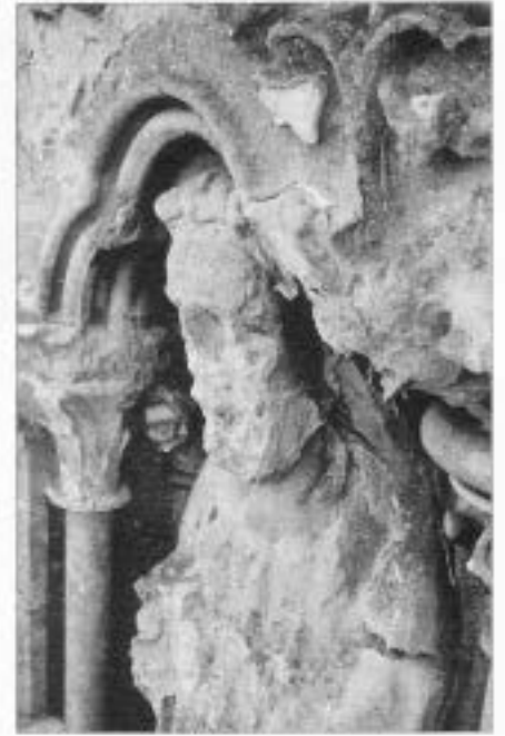
Figure 2 Decayed apostle, Wells Cathedral. The limestone reacts with acidic air pollutants to give salts, which then cause further damage.
