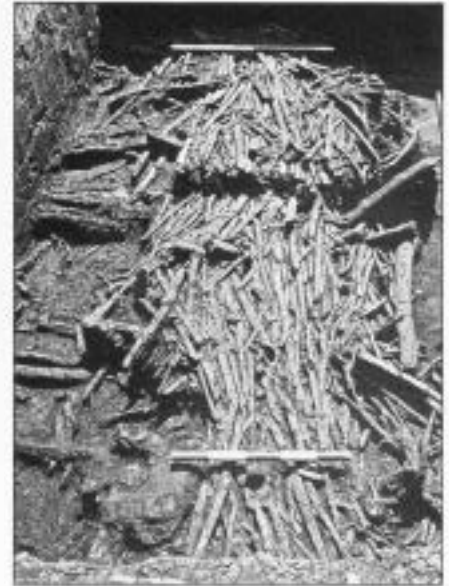
Figure 1 Remains of a Middle Bronze Age trackway found at Beckton, between West Ham and Barking in northeast London; it was built on peat and consisted of a V-shape wooden cradle filled with bundles of alder brushwood.
