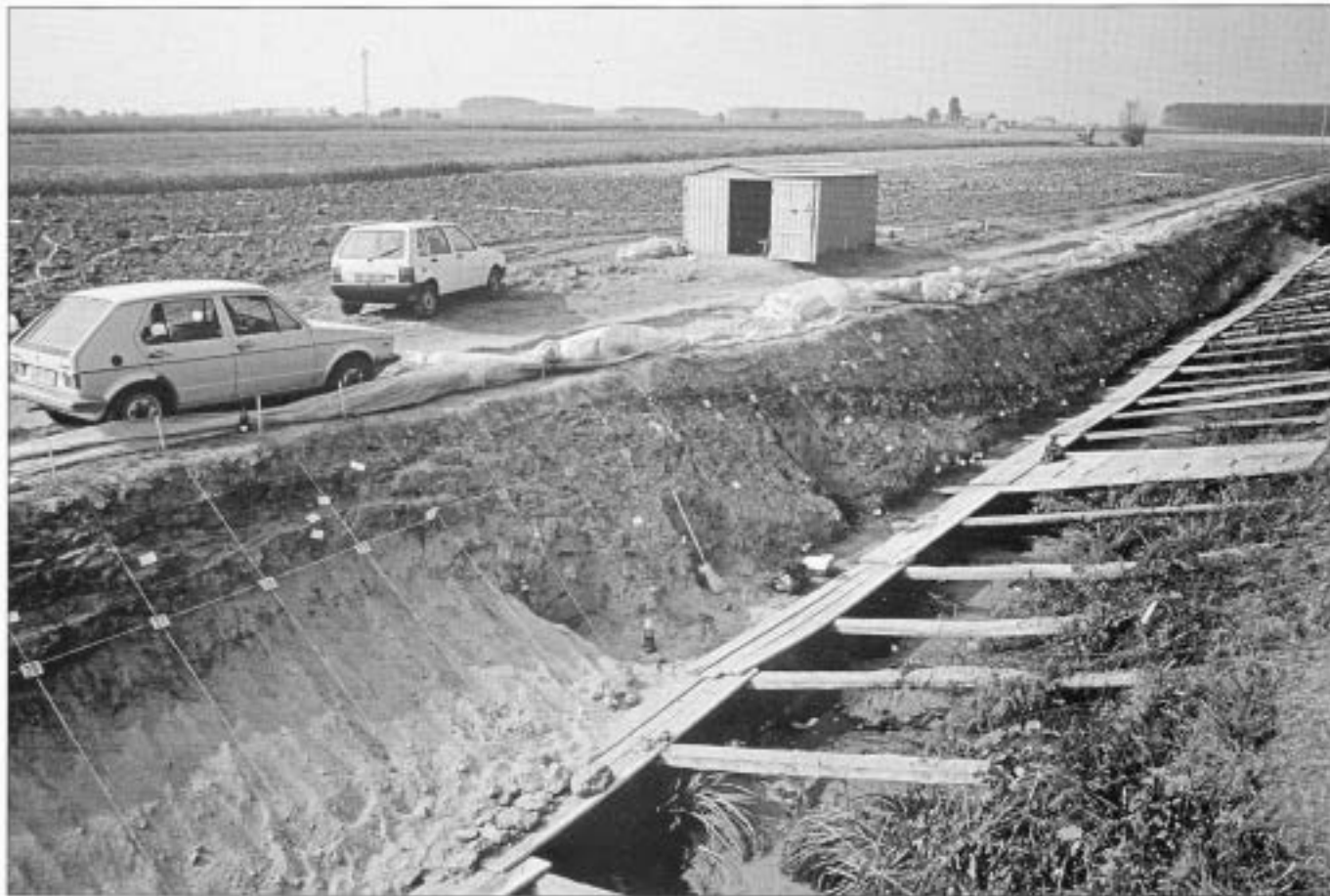
Figure 4 A section (cut by machine for field drainage) through a Bronze Age bank and ditch at the site of Fabbria dei Soci.
