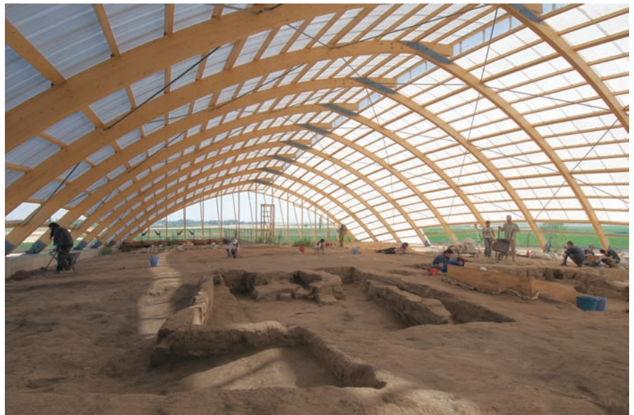
Figure 1 The new shelter constructed in 2008 over the North area of Çatalhöyük (including the 4040 Area); the shelter was designed by Atölye Mimarlık in Istanbul and serves to protect the archaeological remains and to become a display area for the public
