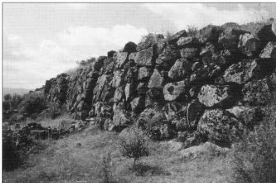
Figure 4 Massive Hittite masonry, 5 m high, at the site of Dumanlı; note the inward slope of the wall face and the vertically stepped façade, features also found in the contemporary walls of Troy VI, Alishar and Hattuša.
